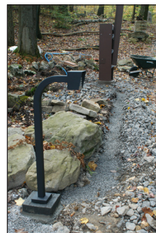
Keypad Foundation & Finished Keypad Assembly
