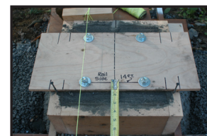
Center to Center of inside anchor bolts = length of rails
