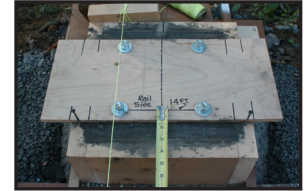
Center to Center of inside anchor bolts = length of rails
