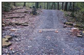
Use a string and level across the road to ensure gate is level after installation (Ref Fig. 1, pg. 3)
