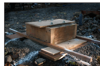
Foundation showing plywood template and wood form
