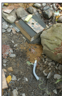
Keypad Foundation & Finished Keypad Assembly
