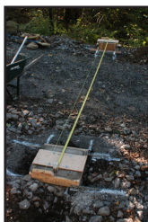
Setting hinge and rest posts relative to rail length
