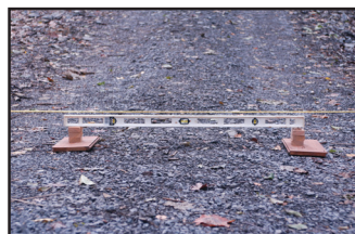
Use a string and level across the road to ensure gate is level after installation (Ref Fig. 1, pg. 3)
