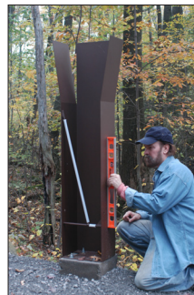
Use a level to ensure that gate posts are plumb
